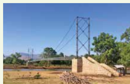
A pedestrian suspension bridge in Ethiopia.
